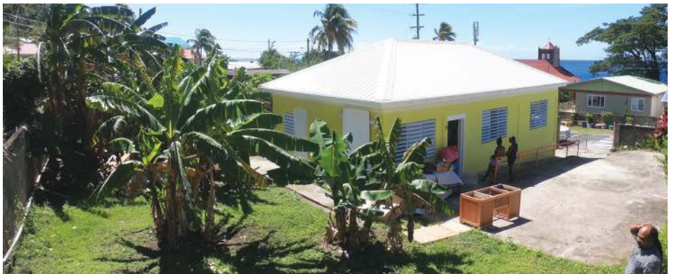
In the aftermath of Hurricane Maria, Americares has rebuilt 11 primary health centers throughout Dominica.
