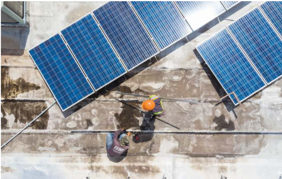
In Puerto Rico, AmeriCares installed solar energy systems to ensure health centers can function if future storms cut power.
