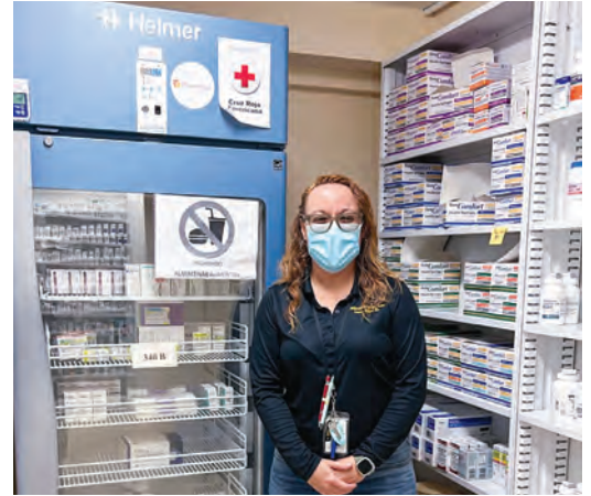
Clinic Administrator Wendy Morales and her staff relied on a solar power system provided by AmeriCares to keep medicine safe and cold after Hurricane Fiona damaged Puerto Rico's power system.
