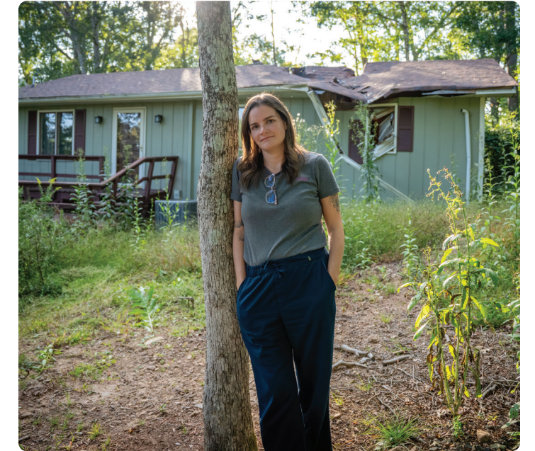
Hannah stands in front of her damaged home in North Carolina.
